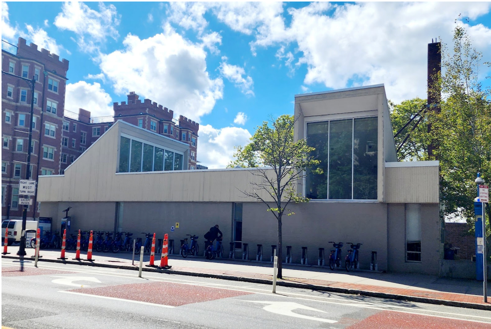
MIT Building W11 (40 Massachusetts Avenue) where CAVS was located.
